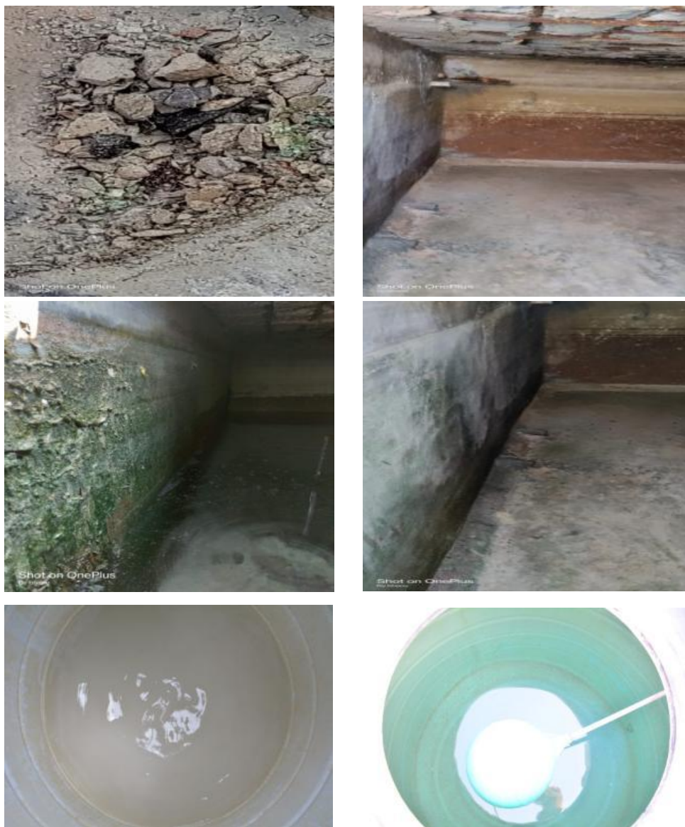
Before and after pictures of water Tank Cleaning activity at LBS block
